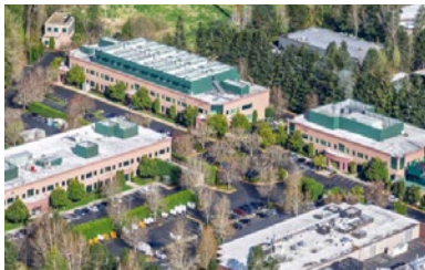
Acquisition (Q3 2025) West Willows Technology Center Other (Data Center); Seattle MSA
