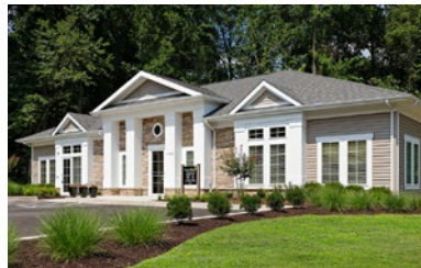
Disposition (Q3 2025) Poplar Glen Apts Multifamily; Baltimore MSA
